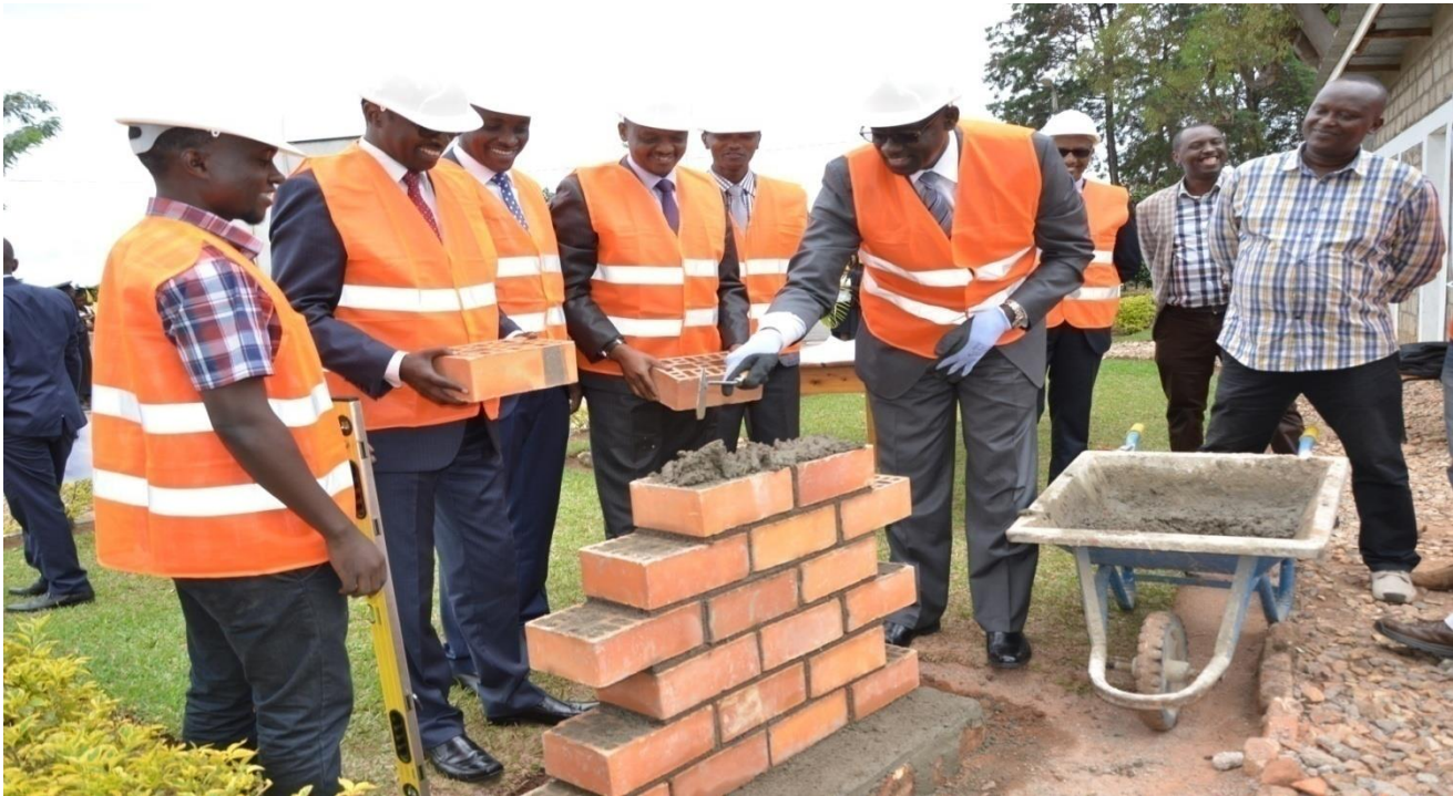
Figure 5: Honourable Minister Johnston Busingye at the lunching of the construction of the Second Phase of ILPD Building on 19th May 2016.
