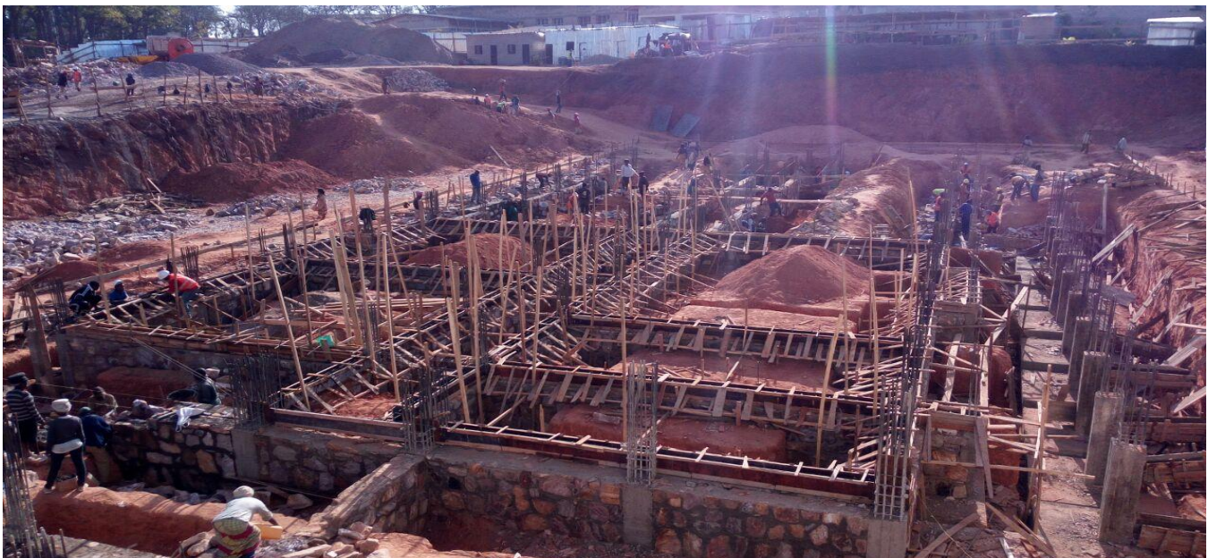
Figure 6: Construction activities of ILPD second phase
