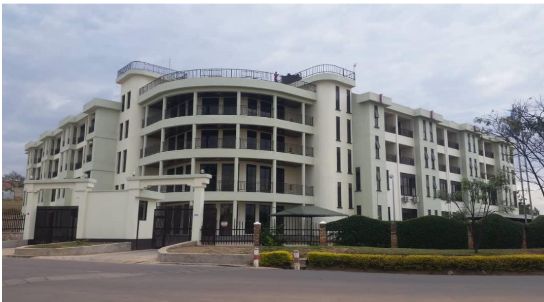
Figure 6: iMutakara Complex completed.
