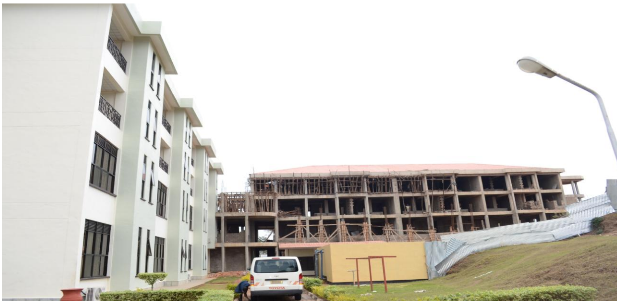
Figure 7: Construction works of ILPD Building second phase
