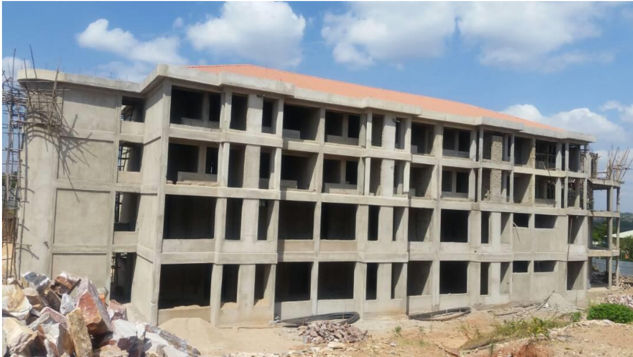
Figure 6: Construction works of ILPD Building second phase
